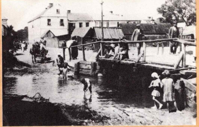
Children often gathered at the town bridge to splash in the water while their mothers washed clothes.
